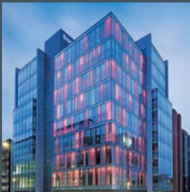
Sentinel Building, Glasgow, Groß- britannien Sentinel Building, Glasgow, Great Britain
